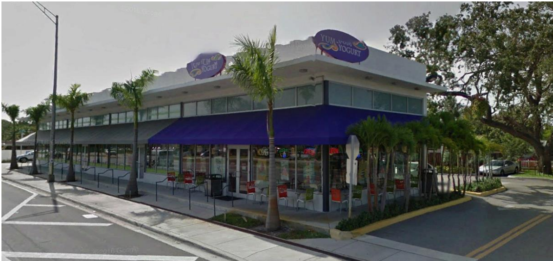
Project Name: YUM-YUM YOGURT STORE Project Location: Miami Design, Drawings, & Calculation MEP by: Bijan Abidian DATE: 2013
