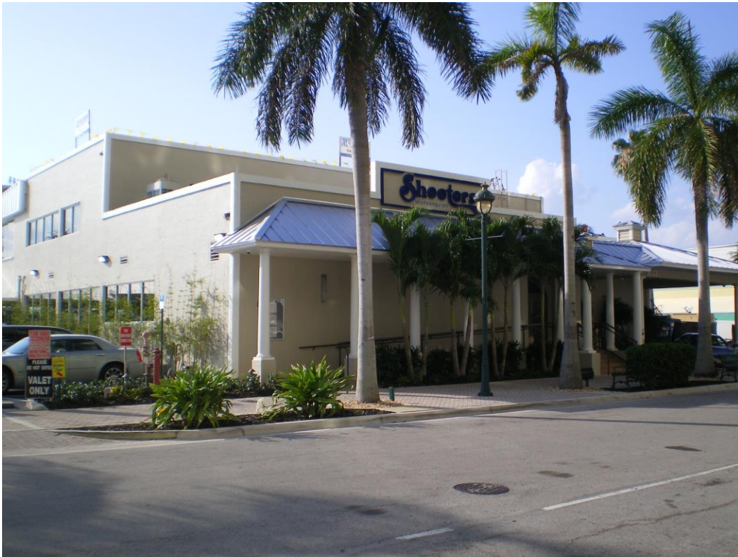
Project Name: Shooters Restaurant Fort Lauderdale, Florida Design, Drawings, & Calculations Structural Remodeling by: Bijan Abidian DATE: 2014
