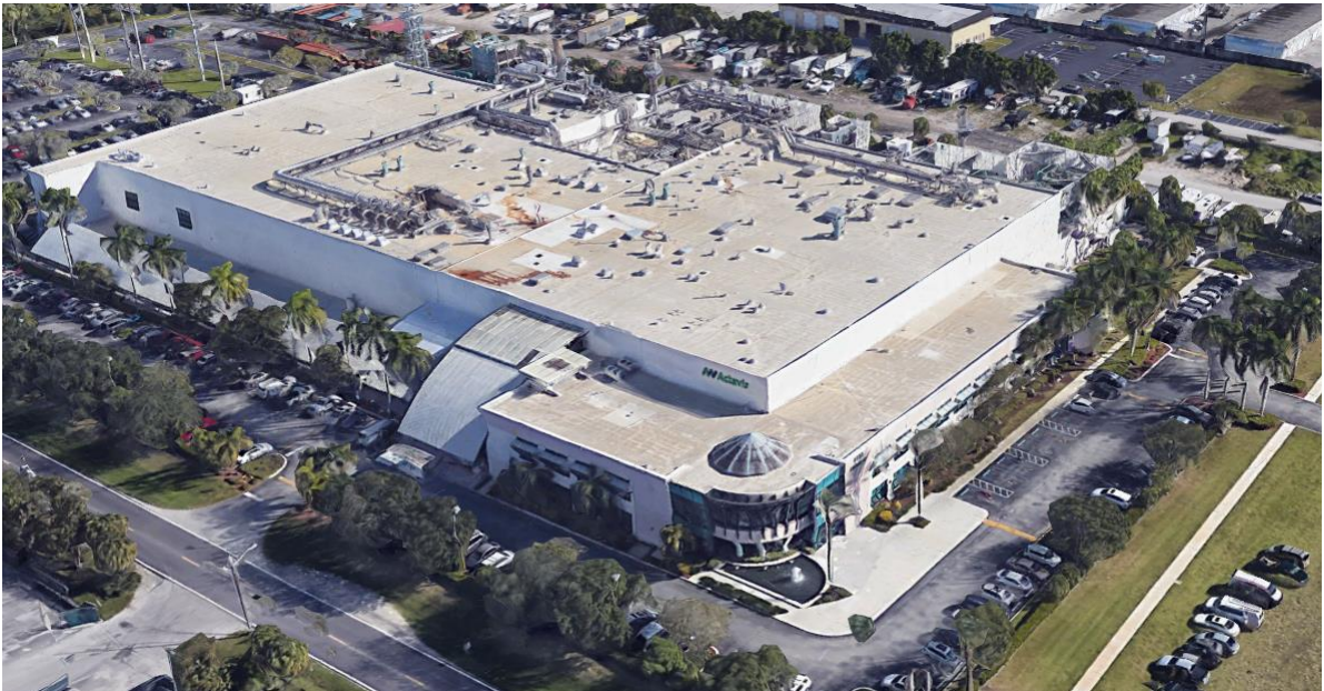
Project Name: ACTAVIS PHARMACY FACILITIES 4955 Griffin Road Fort Lauderdale, Florida Design, Drawings, & Calculation Structural & Mechanical by: Bijan Abidian DATE: 2014
