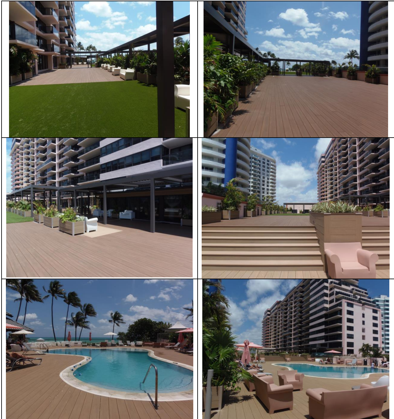
Project Name: Alexander Resort and Hotel Outdoor Pools and Decks Miami Beach Design, Drawings, & Calculation Architectural, Structural, Mechanical, Electrical, and Plumbing By: Bijan Abidian DATE: 2021 and 2022
