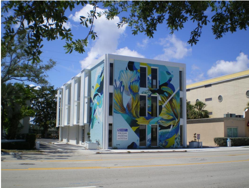
Project Name: Office Building Project Location: Fort Lauderdale Design, Drawings, & Calculations: CE, AE, SE, & MEP by: Bijan Abidian DATE: 2017
