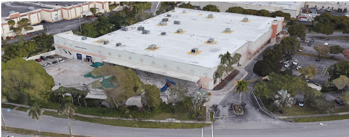
Project Name: Broward Math & Science School Renovation & Remodeling-Interior Alteration 6101 N.W. 31 st Street Margate, FL 33063 General Contractor: Blue Ocean Construction, Inc. Design, Drawings, & Calculation CE, AE, SE, & MEP by: Bijan Abidian DATE: 2016-2017
