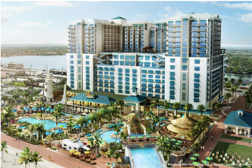
Project Name: Margarita Ville Hollywood Beach Hollywood Beach, Florida Design, Drawings, & Calculations all outdoor Tiki structures by: Bijan Abidian DATE: 2015-2016
