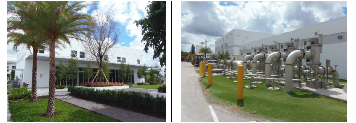
Project Name: NSID RECORD BUILDING 9700 NW 52th Street Coral Springs, FL 33071 Design, Drawings, & Calculations Civil-Architectural-Structural-Mechanical-Electrical-Plumbing by: Bijan Abidian DATE: 2021
