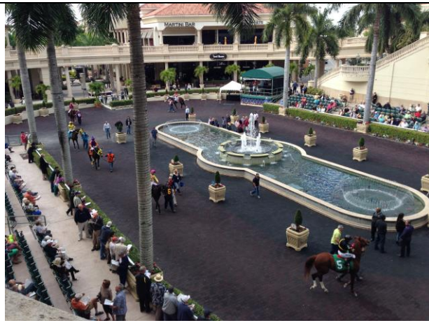
Project Name: Gulfstream Park-Walking Ring Platforms Project Location: Hallandale Beach, Florida Design by: Bijan Abidian Design, Drawings, Calculation SE, & MEP: Bijan Abidian DATE: 2013-2014
