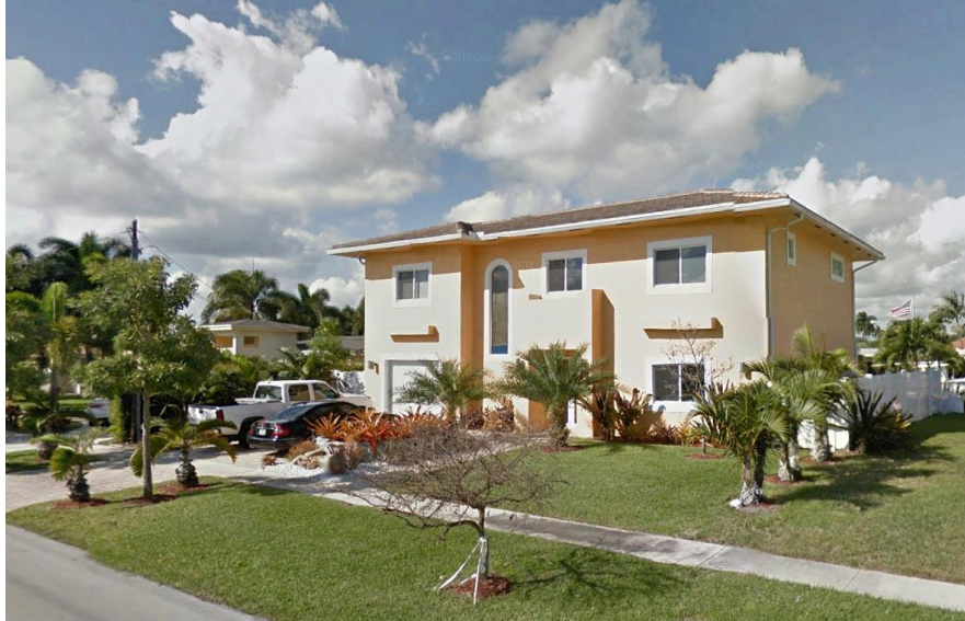
Project Name: 341 SE 12 th Street Project Location: Pompano Beach Design, Drawings, & Calculation CE, AE, SE, & MEP by: Bijan Abidian DATE: 2011
