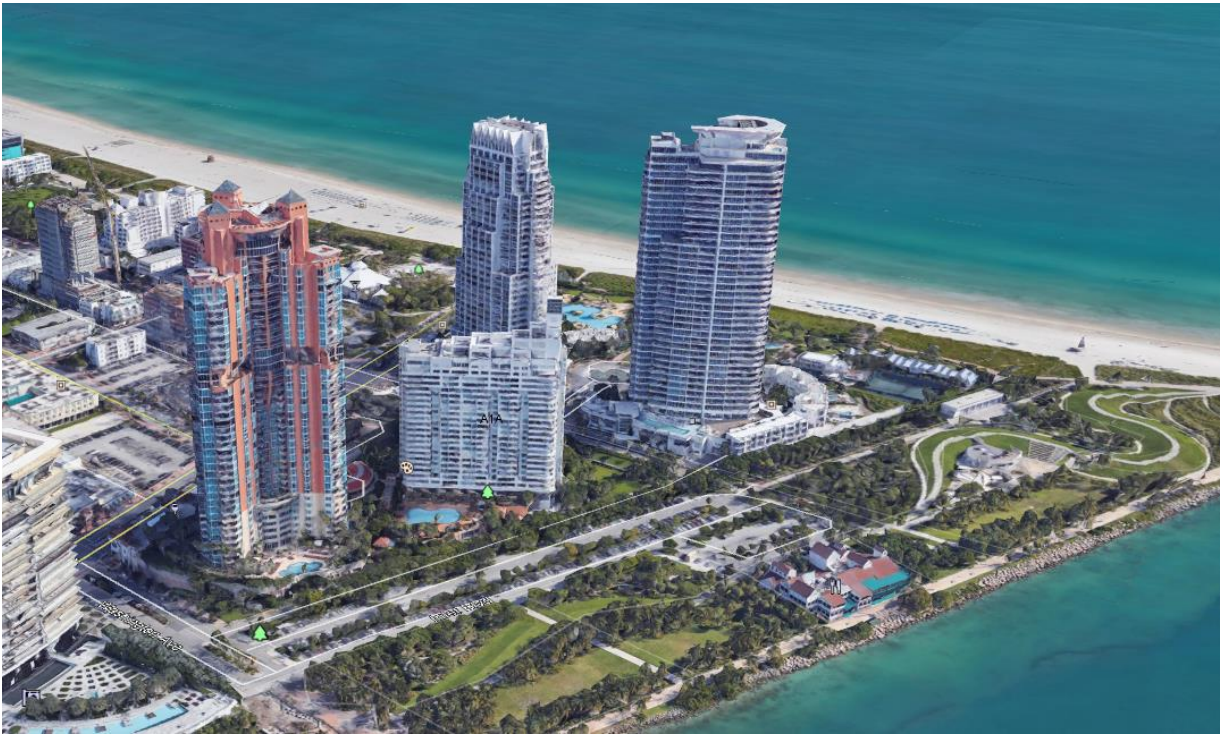
Project Name: PORTOFINO + SOUTH POINT TOWER 300 South Point Drive Miami Beach, FL 33139 Design, Drawings, & Calculation CE & MEP by: Bijan Abidian DATE: 2017-2018
