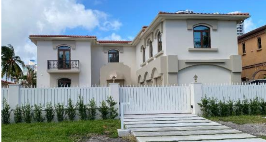
Project Name: Sunny Isles Beach Residence 18950 North Bay Road Sunny Isles Beach, FL 33160 Design, Drawings, & Calculation CE, AE, SE, & MEP by: Bijan Abidian DATE: 2016-2019
