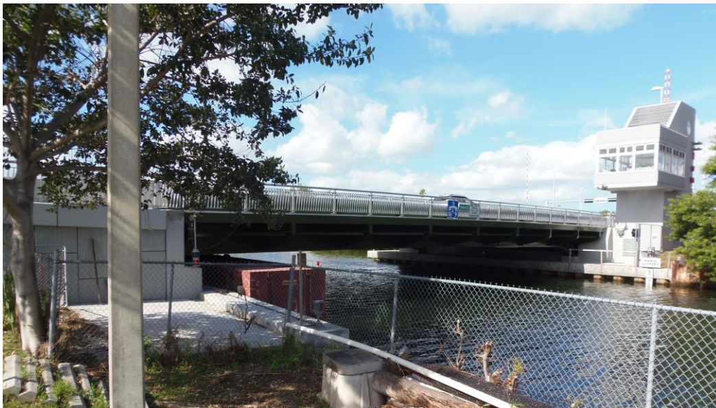
Project Name: Tamiami Trail Bridge Miami, Florida Design, Drawings, & Calculations Sewer Systyem by: Bijan Abidian DATE: 2018
